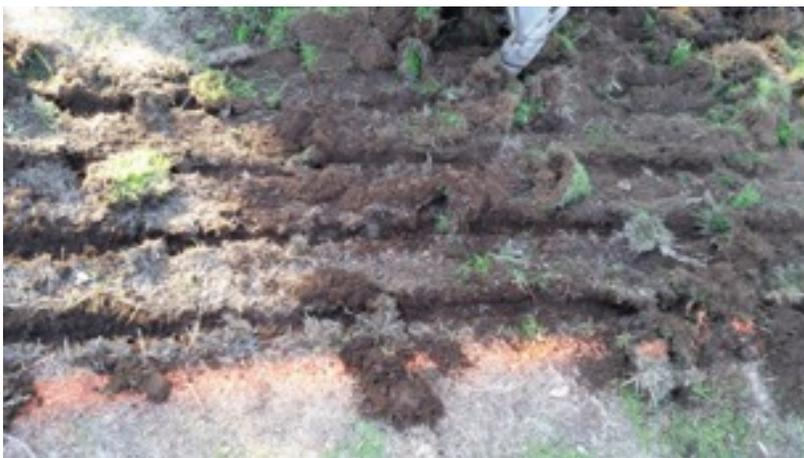
Apply the base layer of sand media as per the design. The top of sand layer under the coil must be level.
