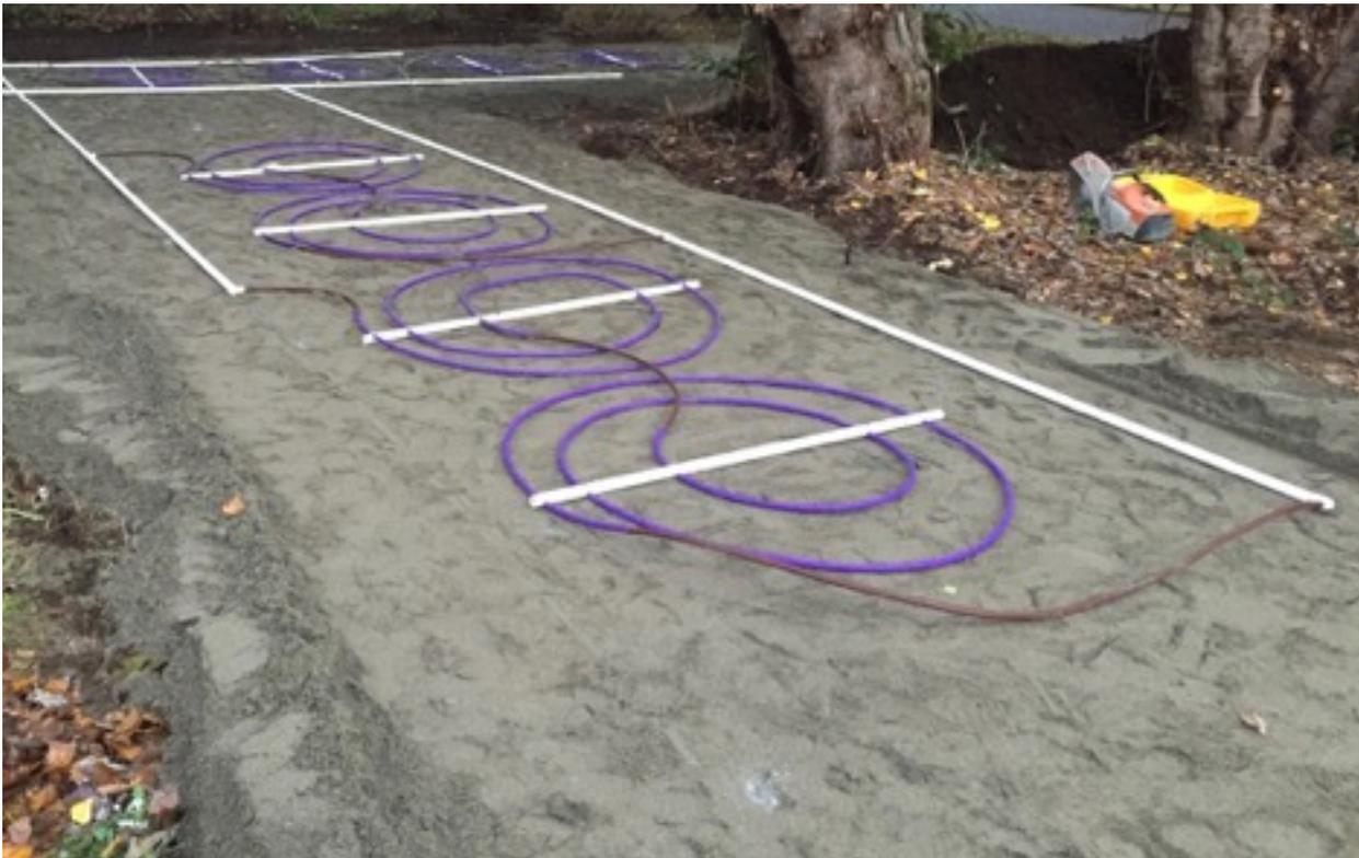
Place the coils and connect the supply and flush manifolds as prescribed in the design.
